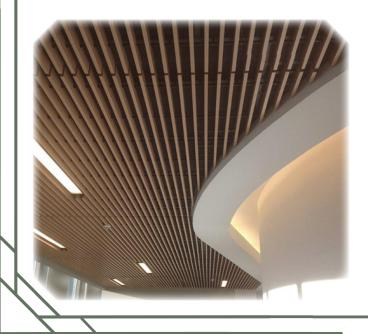
The RB Baffle system blades are easily installed onto the runners with drywall screws and can be attached to walls using sheathing or furring strips.
