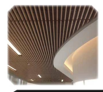
The Dowel Rod Backer panels are factory assembled with wooden dowels at 12" O.C. Dowels are typically painted flat black - but custom finishes are avaailable per project specifications.
